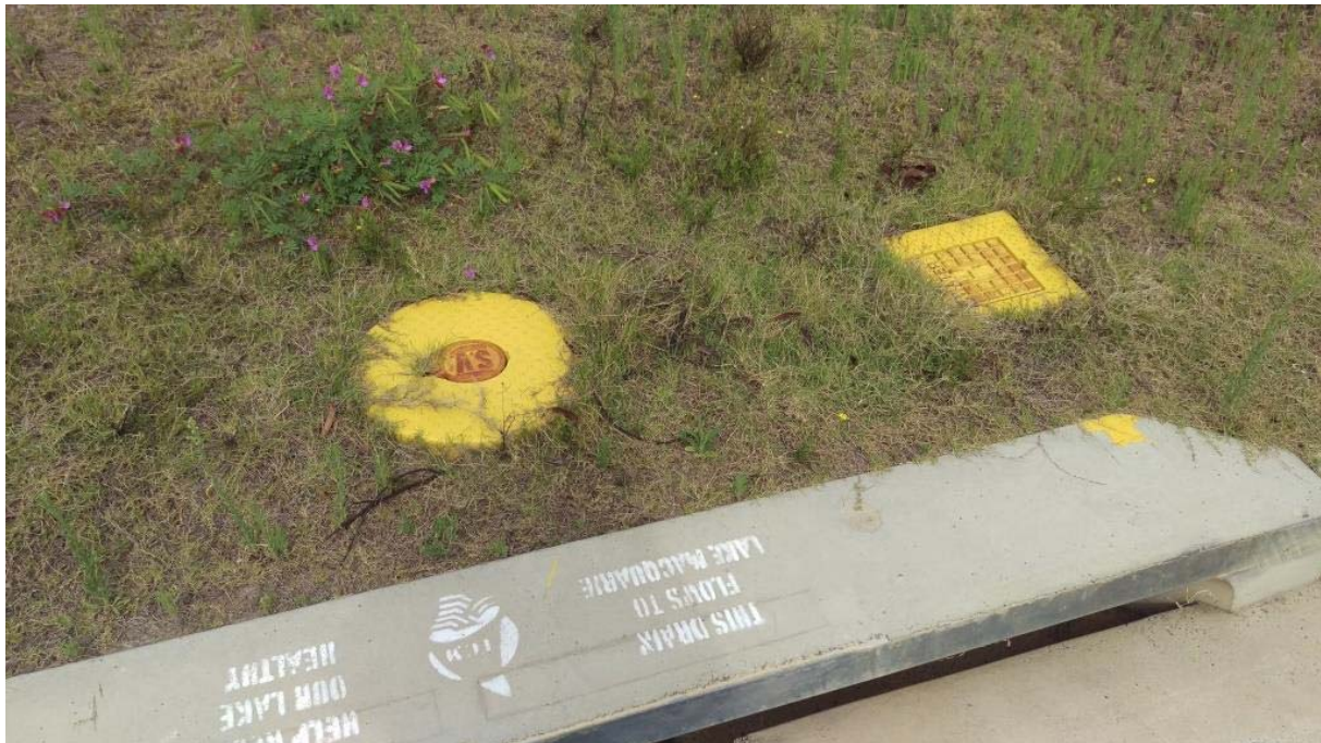
Figure D.3.2 Colour coded valve and hydrant covers –covers and surrounds coloured yellow for potable (drinking) water.
