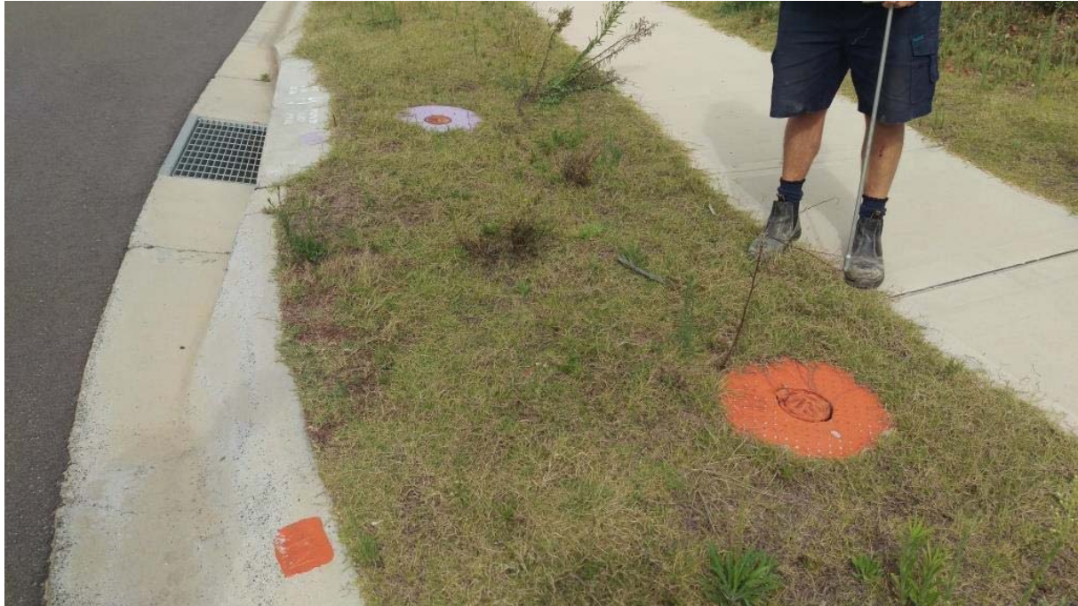
Figure D.3.1 Colour coded valve covers – surround coloured lilac for recycled water with embossed labelling “RECYCLED”; cover and surround coloured orange for pressure sewer.
