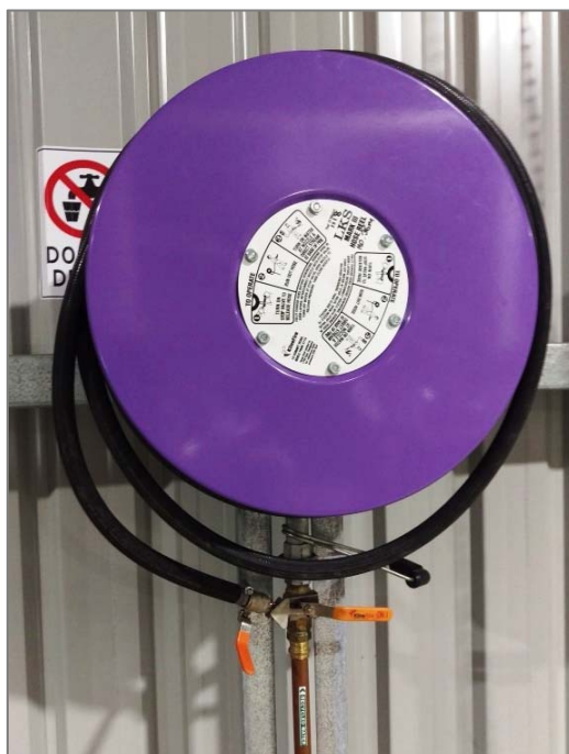
Figure A.5.5 Service water installations are appropriately colour coded. Note signage in the background.
