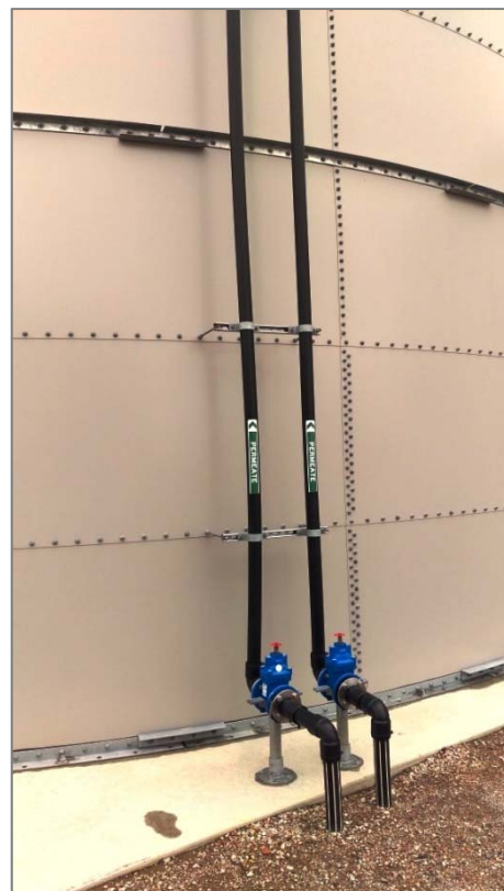
Figure A.5.4 Pipework labelling and colour coding – blue striped for potable water and cream striped for MBR permeate.
