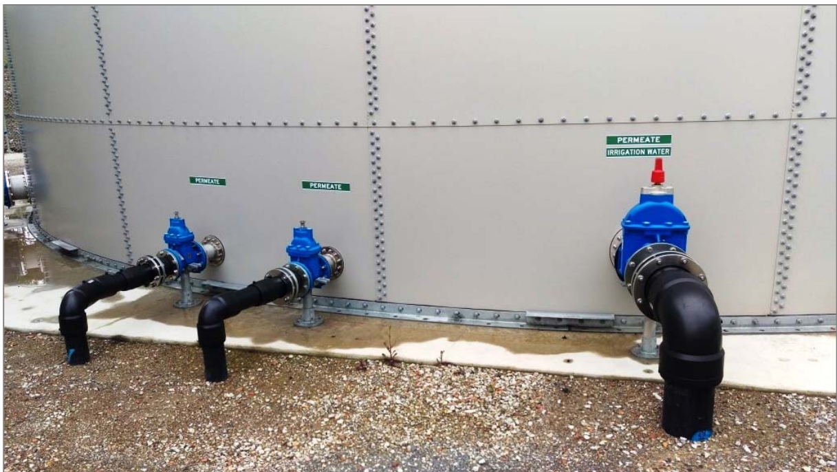
Figure A.5.8 Extensive labelling is in place on all tank connections (for example).
