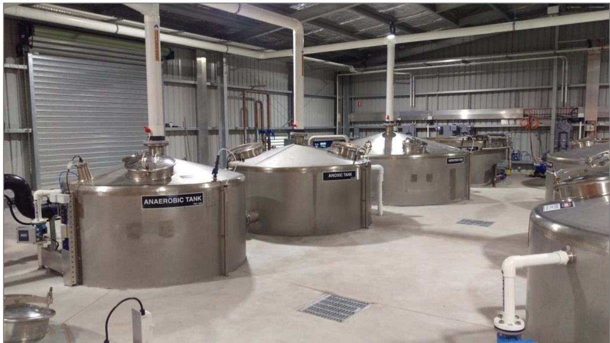
Figure A.5.1 MBR process tanks (anaerobic, anoxic and aeration) where gas is produced are fully enclosed with positive extraction of gases through an odour scrubbing unit.
