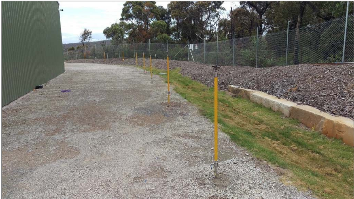
Figure A.5.3 Fire sprinkler system between the treatment plant building and bushfire threat (bushland).
