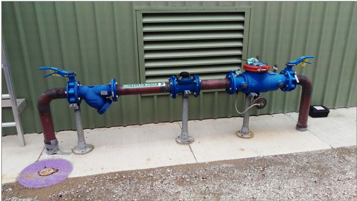
Figure A.5.9 Backflow prevention.
