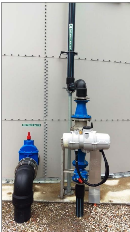
Figure A.5.4 Pipework labelling and colour coding – blue striped for potable water and cream striped for MBR permeate.
