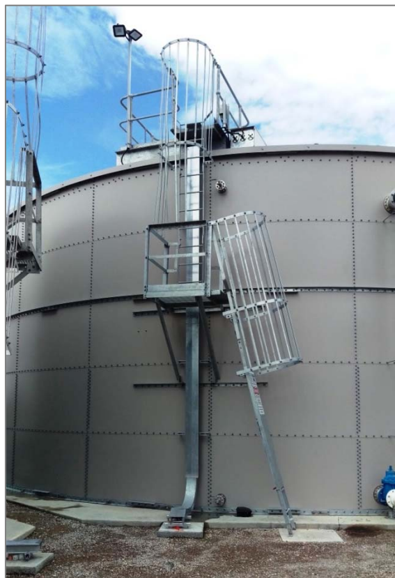
Figure A.5.10 Roof access ladders fitted with safety cages and lockable gates.
