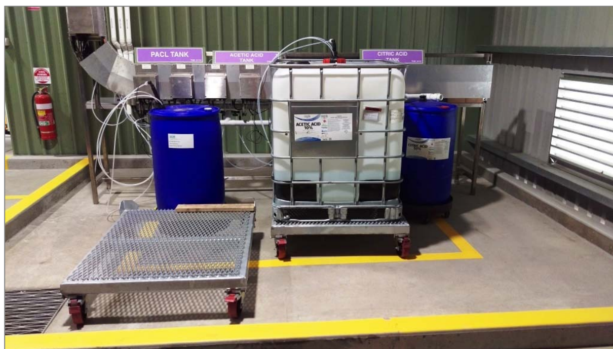
Figure A.5.6 Bunded chemical dosing area; dosing pumps in background.
