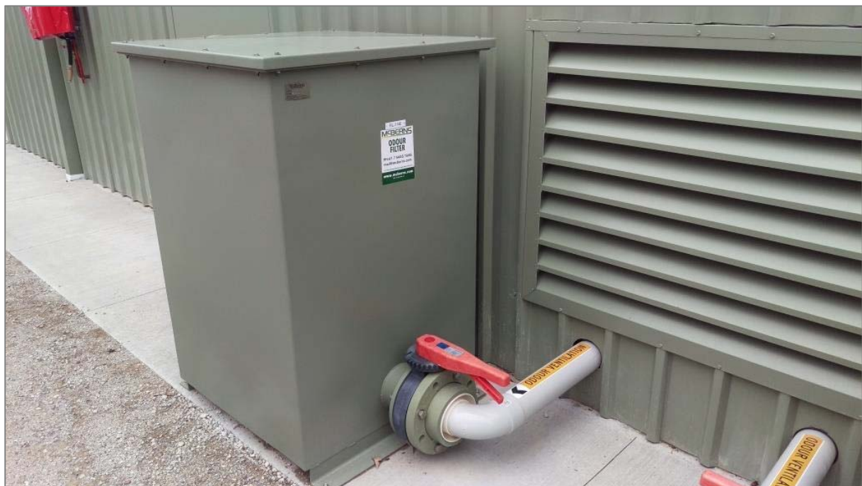
Figure A.5.2 McBerns odour scrubbing unit (filter) located adjacent to the treatment plant building.
