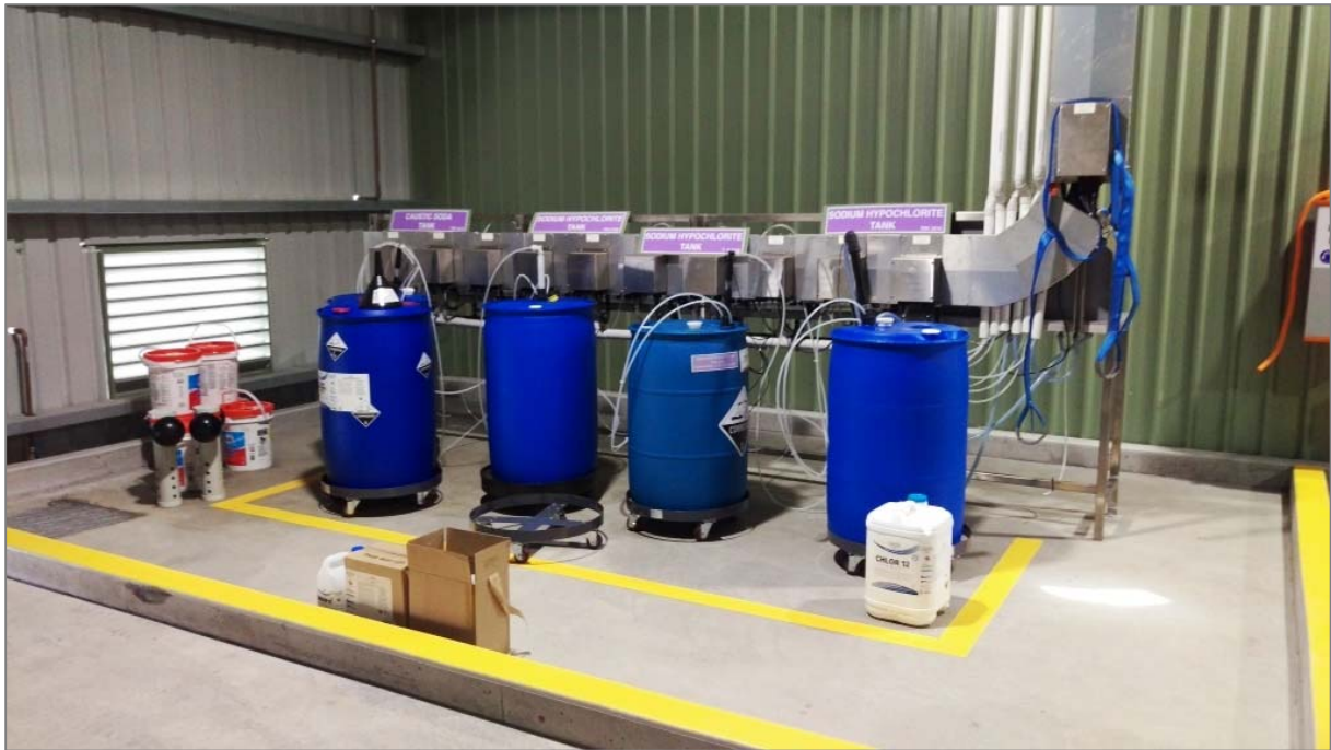
Figure A.5.7 Bunded chemical dosing area; dosing pumps in background.
